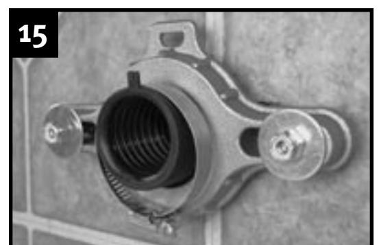
Install the gear clamp with the screw head at the bottom, but do not tighten.
