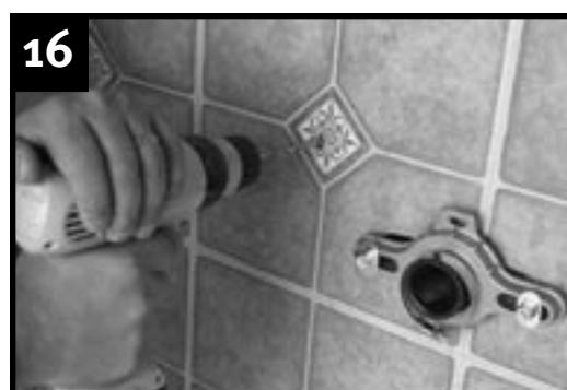
Drill holes for the lower anchor screws and insert plastic anchors.
