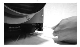
When service is complete, initiate a call for dehumidification and check that the compressor and fan activate. If using the VisionPRO IAQ or TrueIAQ controls, reset maintenance reminders.
